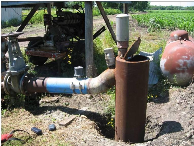
Figure 55. Riser sampler on irrigation pipe at the Mark Verstuyft Well. This structure was built for the purposes of this study.
