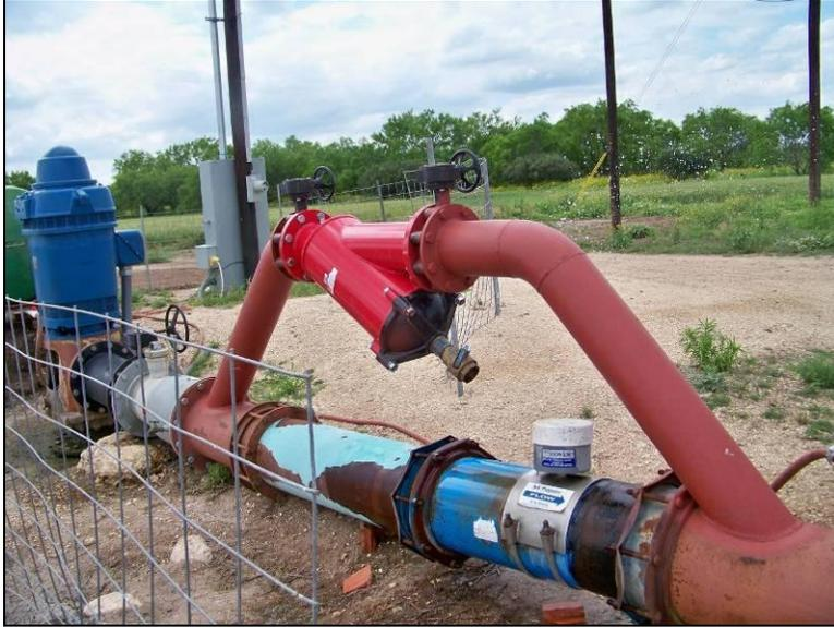
Figure 5. In-line filter sampler.
