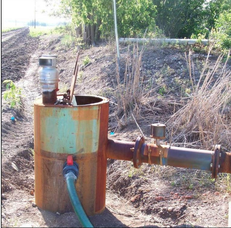
Figure 63. A closed riser sampler was installed at the Raymond Wauters Well in 2010.
