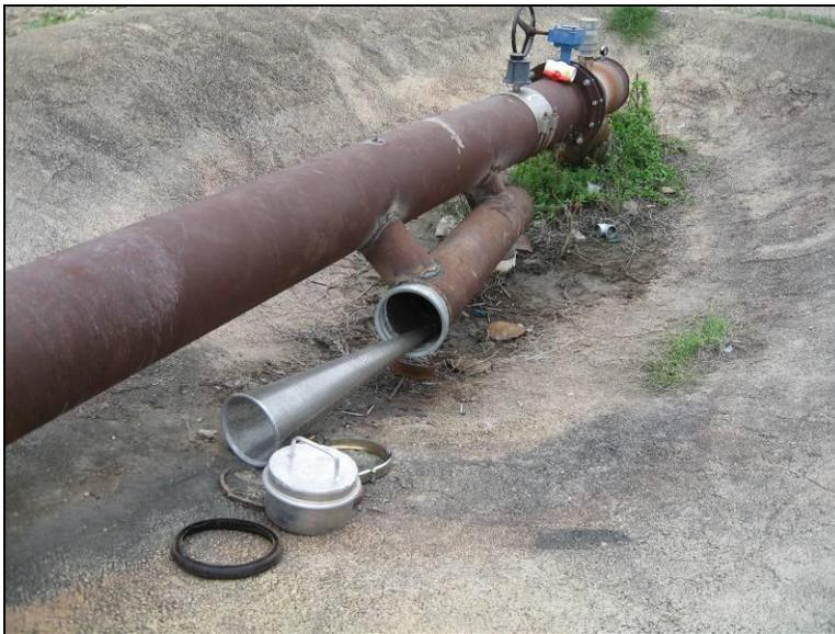
Figure 89. A filter style sampler was installed on the aqueduct outflow at Verstuift Farms to facilitate easier sampling. The filter is shown here in its disassembled state.
