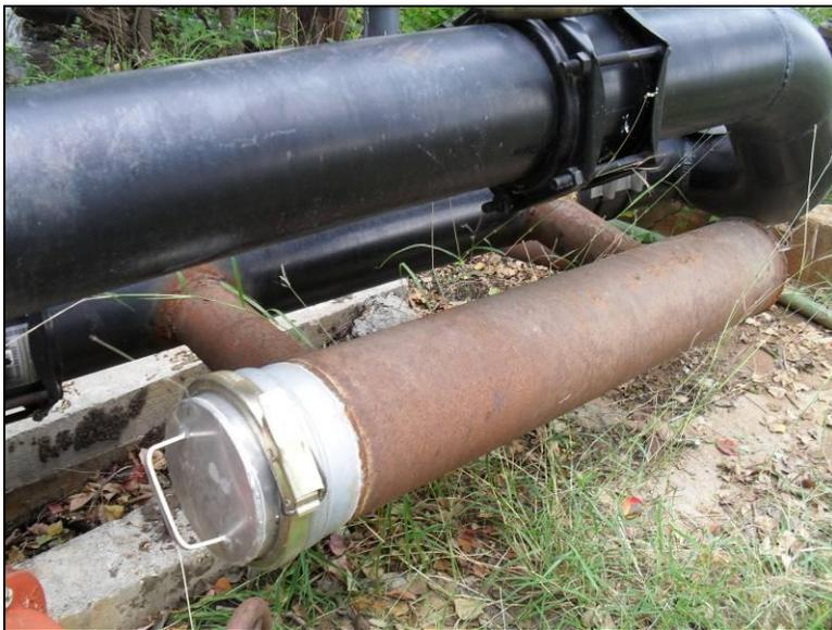
Figure 91. The modified sampling setup at the Verstuyft Home well involved detouring the water to run through a filter that could be sampled before the water returned to the main irrigation line.
